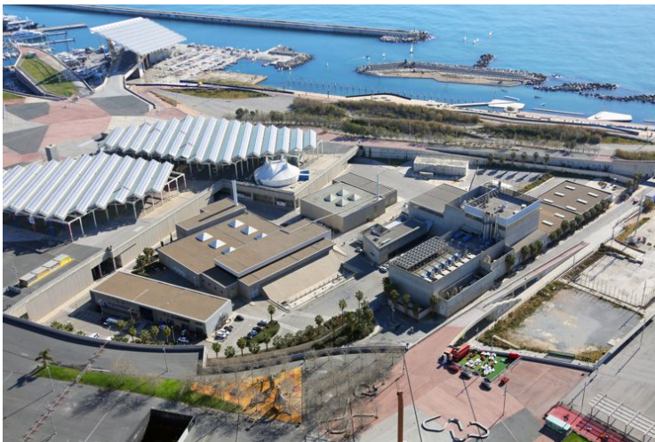
Besòs Wastewater Treatment Plant (Barcelona)
