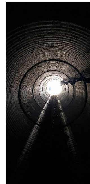
Detalle interior hinca
