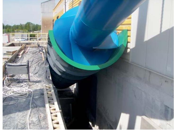
inserting the turbine into the modified channel
